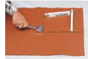
Using ordinary tools, measure the appropriate width required to seal the abutment
