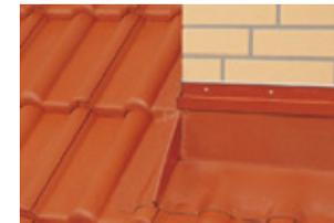
Apply a Connection Strip securely with non-corrosive screws to the upper edge of Wakaflex, sealing off with Coverfill between the wall and Connection Strip
