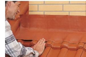
Then release the butyl strip on the tile side and mould onto the clean tile surface
