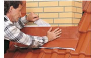
Release the butyl strip against the wall first ensuring a straight line along the wall
